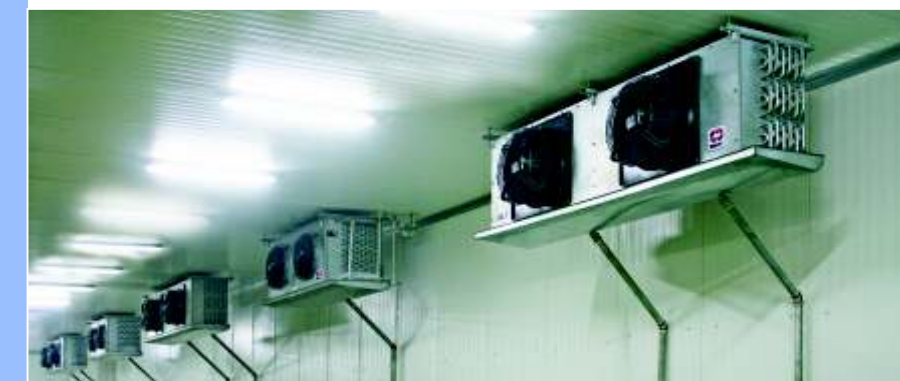
Spiral Freezer Ammonia Unit Cooler AND-S Capacity Range 28.6 to 365.9 kW Fan Diameters 630 or 710 mm No of fans 2, 3, 4 or 5 Fans Fin Spacing 6, 8, 10, 12, 15 or 12/15
