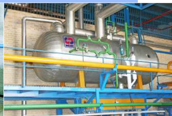
Ammonia Receiver NRC Diameter Range up to 2 m Length Range up to 12 m Temperature Range -10 to 50°C Working Pressure Range up to 20 bar
