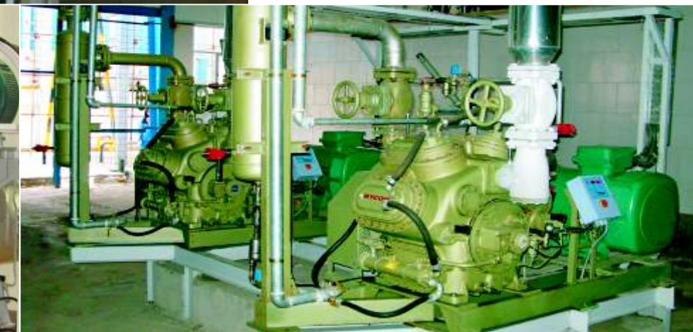
MAYEKAWA Reciprocating Chillers Capacity Range 41 to 677 kW Refrigerant: Ammonia or Freon Temperature Range +12 to -30°C
