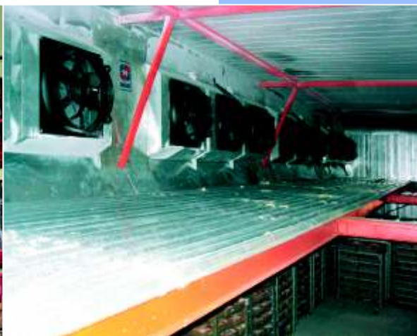
Tunnel Freezer Ammonia Unit Coolers AND-T Capacity Range 48 to 295kW Fan Diameter 630 or 710 mm No of Fans 2,3,4 or 5 Fans Fin Spacing 6, 8, 10, 12, 15, or 12/15
