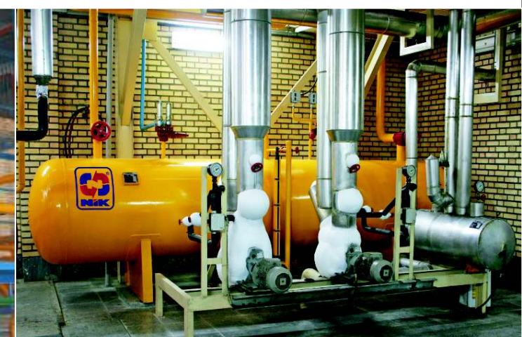
Ammonia Surge Drum NSD Diameter Range up to 1 m Length Range up to 3 m Working Pressure Range up to 20 bar
