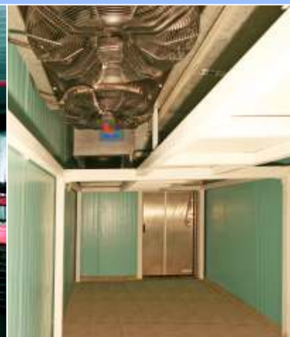
Angle Type Ammonia Unit Cooler AND-A Capacity Range 48 to 203.3 kW Fan Diameters 630 or 710 mm No of fans 2, 3, 4 or 5 Fans Fin Spacing 6, 8, 10, 12, 15, or 12/15
