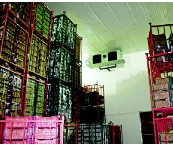
Tunnel Freezer Ammonia Unit Coolers AND-T Capacity Range 48 to 295kW Fan Diameter 630 or 710 mm No of Fans 2,3,4 or 5 Fans Fin Spacing 6, 8, 10, 12, 15, or 12/15
